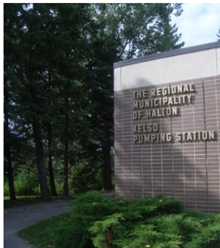
Figure 2: Kelso Drinking Water System Pump Station
