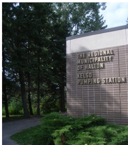
Figure 2: Kelso Drinking Water System Pump Station
